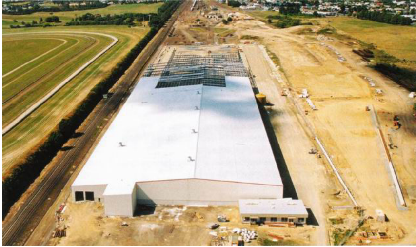
Figure 7: Aerial View of Site under Construction.
