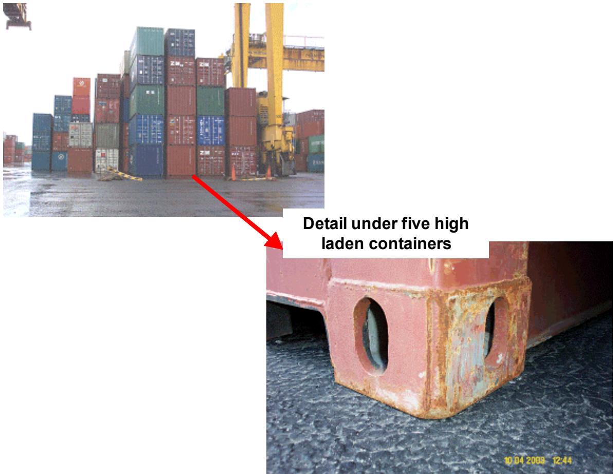
Figure 6: Static loads from container corner castings can exceed 25 MPa.
